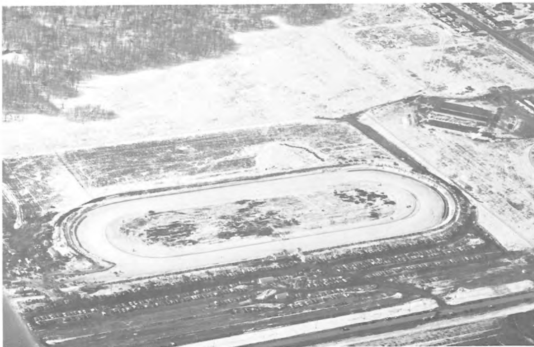
The existing C.P.T.C. Race Complex.
